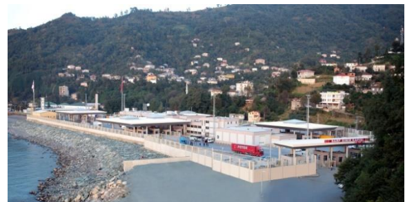
Photo 15 – Sarp BCP after Modernization (2012)
