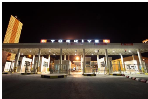
Photo 16 – Sarp BCP after Modernization (2012)
