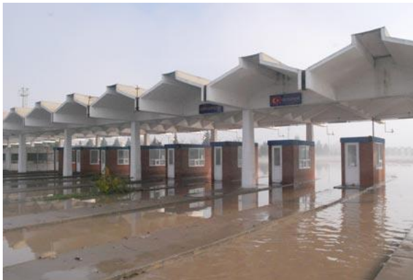
Photo 1 – Kapikule BCP flood (2007)
